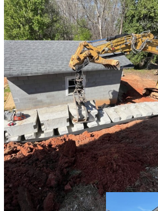
Building of a Retention Wall
